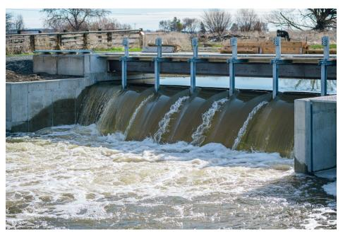
Pictured: The new Sweek Dam on the Silvies River completed fall of 2019 helps ensure efficient management of snowmelt waters reaching Harney Basin flood irrigated meadows. Photo by Jeremy Hill.
