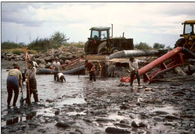
Figure R-21. In 1992 Refuge staff made a huge effort to drain Headquarters Pond with two Crissafulli pumps to remove carp.
