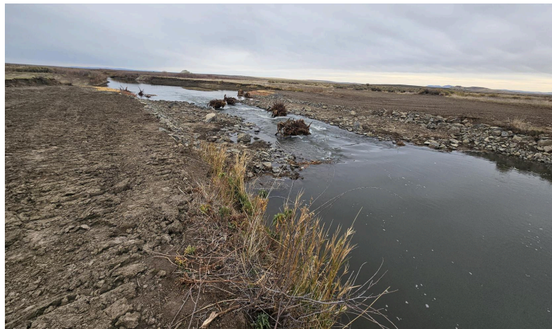
Pictured: The Dunn Dam rock chute mimics the natural stream morphology with a roughened channel.
