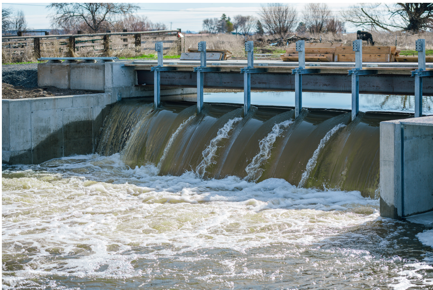
The new Sweek Dam along the Silvies River completed fall of 2019. Photo by Jeremy Hill, jhillimages.com.
