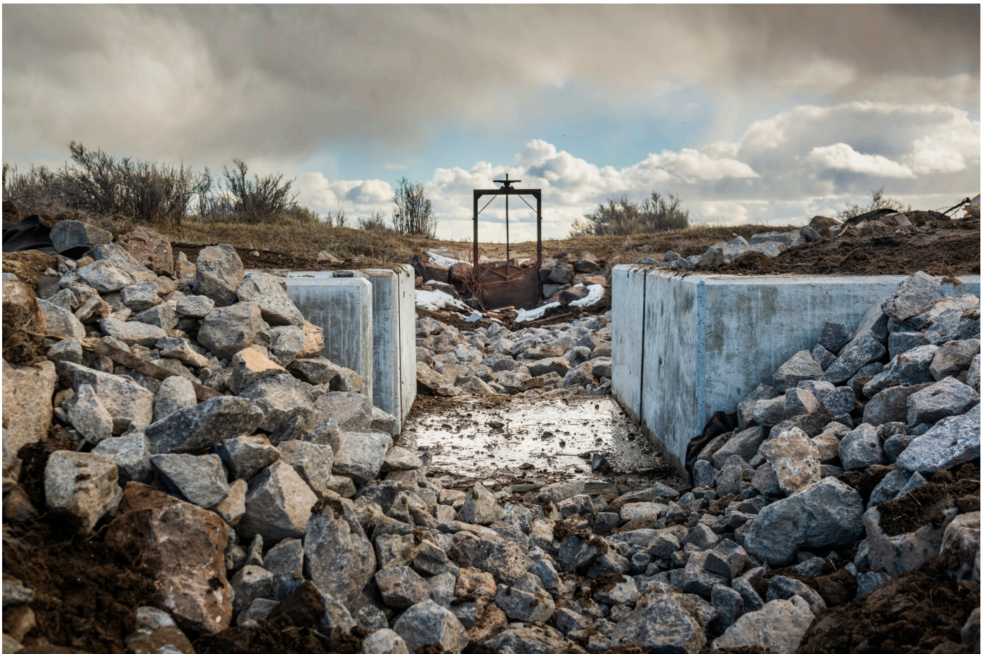
A new concrete diversion structure to more effectively move water to the head gate in the distance. The head gate can be opened as needed to flood the meadow with water that lies beyond the gate. Photo by Jeremy Hill, jhillimages.com.
