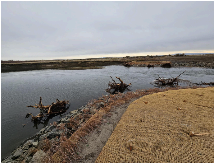
Pictured: The new rock chute that replaced the Dunn Dam mimics natural stream flow and provides fish passage.
